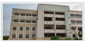
SBS Extension: Structure completed, False ceiling, expansion joint, aluminum work, Sanitary work, electrical work, HVAC work is in progress s. About 78.60% of building work completed.
