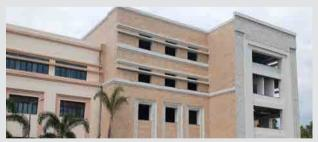
SIF Extension: Structure completed, finishing work such as painting, Aluminum work, false ceiling work, Sanitary work, HVAC & electrical work is in progress. About 75.25 % of building work completed.
